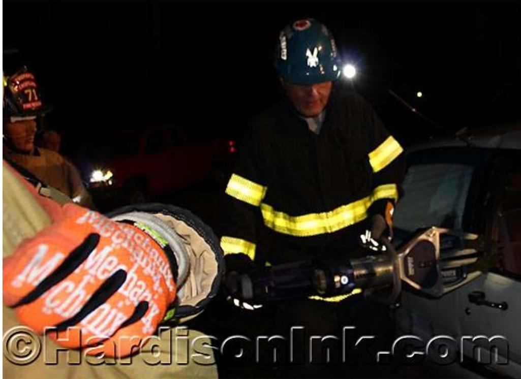
Rest the tool here. Turn this knob. Let the tool work. Tom Winkler reminded firefighters they do not need to force things, because as much as they may think smashing a battery into the tool is the best method, it is not. If the battery is not going into the tool, it is because there is something in the way, like a piece of glass. It is best to store batteries in the tools or in the chargers, he said.
