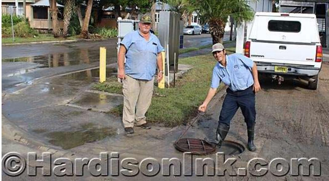
James McCain (left) and Billy Quinn of Cedar Key Water and Sewer Service, check a storm drain pipe. Quinn is replacing the manhole cover here.
