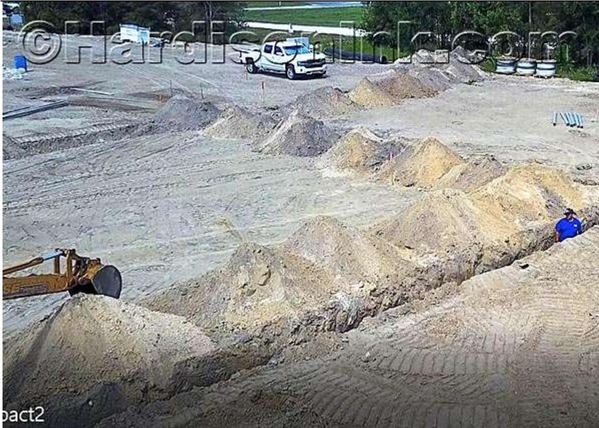
**A worker stands in a deep trench created for developing part of the infrastructure of the RV park. The trench was created by a backhoe, however workers with shovels are needed for some of the finer points of construction on the bottom of the trench. when laying pipe for water and sewer service, one of the many rules of physics that must be applied by builders is that water does not flow uphill -- unless there is pump involved.**
